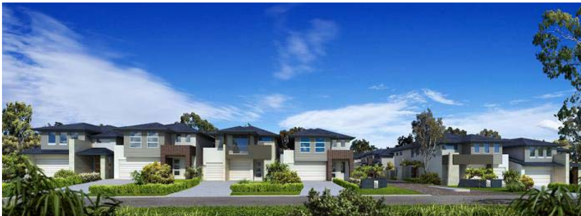
Above: Fairway Gardens, Kellyville
