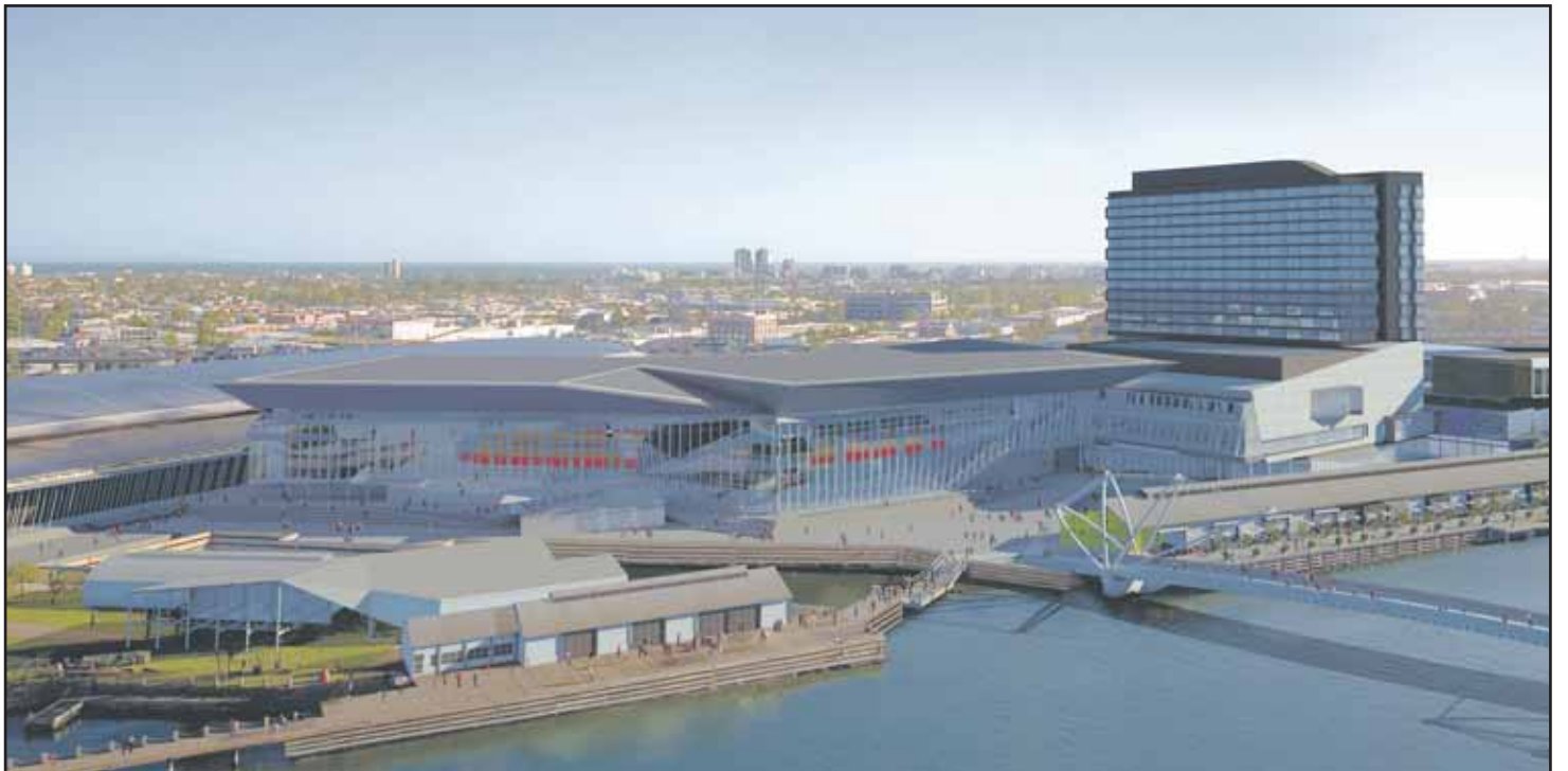
The six-Green Star rated Melbourne Convention Centre, which opens next year, is a prime example of Australia's highly sought-after sustainable construction.
